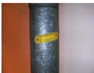
Figure 43 Metal clad gas flue containing chrysotile lining
