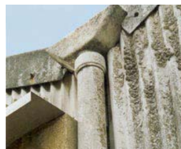
Figure 35 Asbestos cement downpipe
