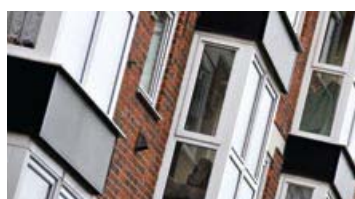
Figure 16 AIB exterior painted panel
