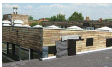
Figure 23 AIB fascia panels with wood effect finish
