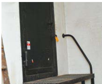
Figure 45 'Durasteel' composite steel and asbestos fire door
