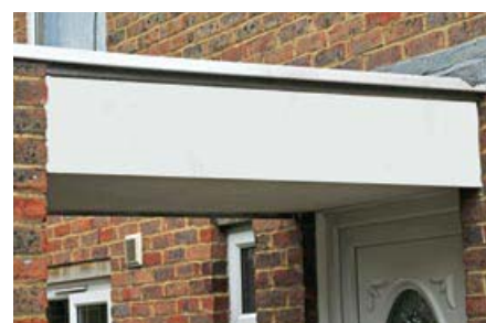
Figure 15 AIB panel in porch
