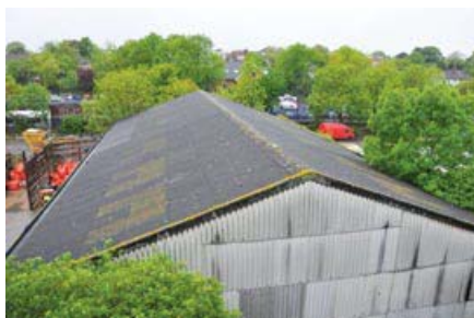
Figure 32 Asbestos cement roof and cladding
