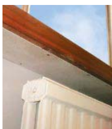
Figure 20 AIB panel between radiator and window
