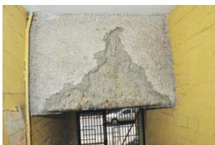
Figure 8 Sprayed coating on building passageway
