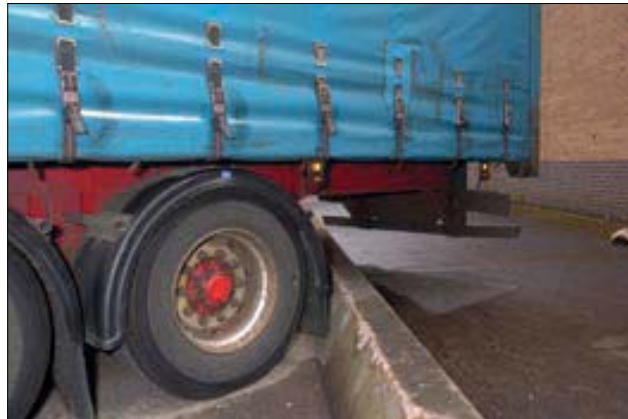
Figure 7 Concrete wheel stop
