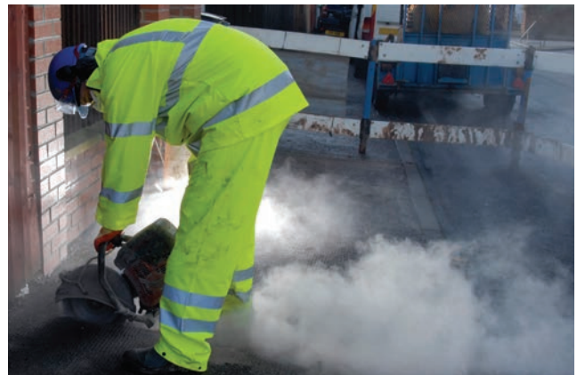
Figure 1 Common tasks like cutting can create very high dust levels
