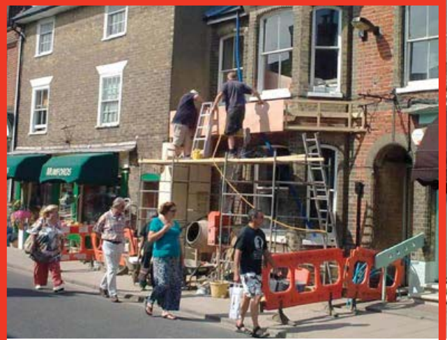
Pedestrians are forced to walk in the road and are at risk from falling tools and materials, and workers are at risk of falling
