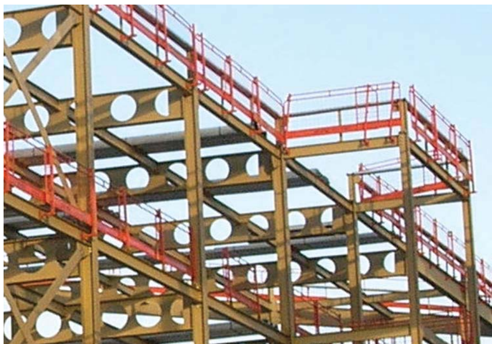
Figure 28 Edge protection installed with the steelwork
