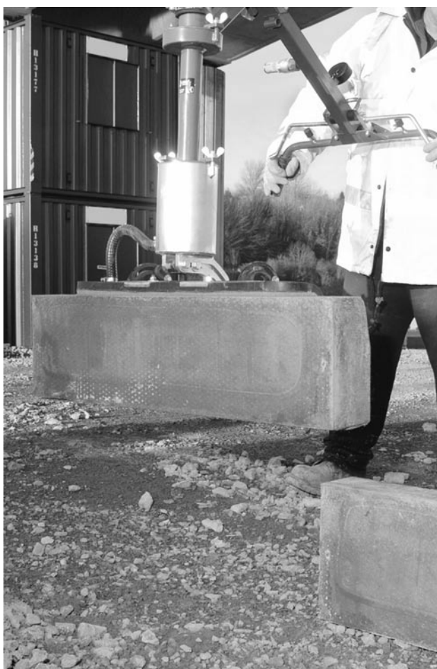
Figure 38 Handling kerbs using a vacuum lifter
