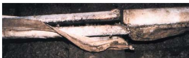
Figure 48a Asbestos-insulated water pipes showing evidence of maintenance work damage, with detached preformed sections and calico wrapping
