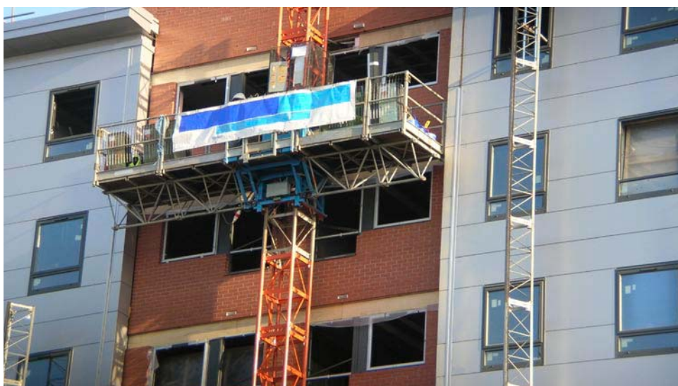
Figure 14 A mast climbing work platform
