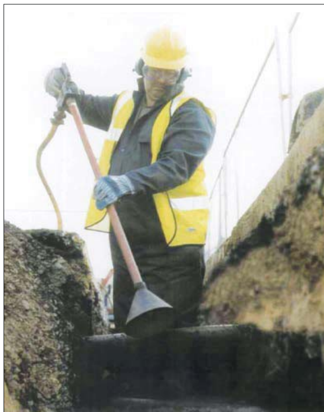
Figure 1 Using an air digging tool
