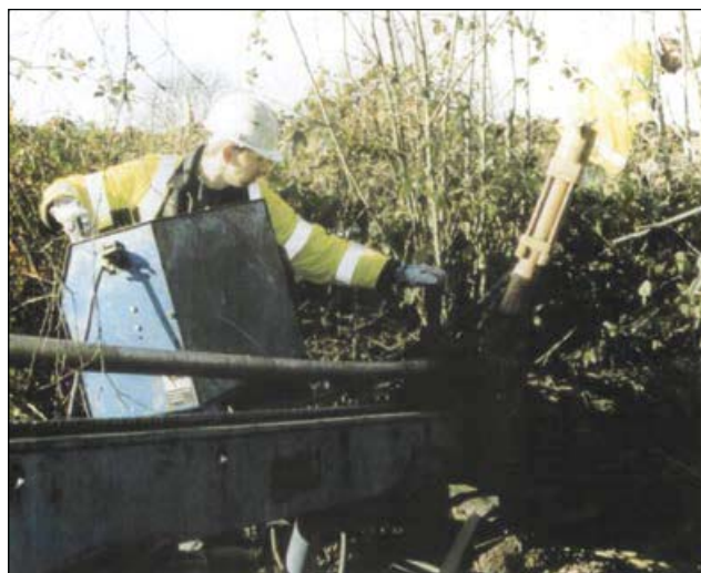
Figure 1 Horizontal drilling being used for laying a cable under a road
