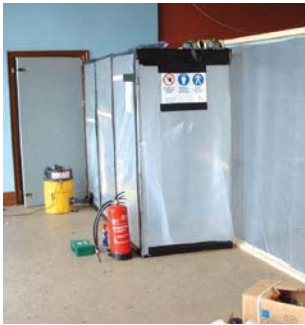
Figure 6.7 An airlock used in transiting
