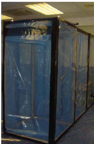
Figure 6.12 Flap arrangements for airlocks
