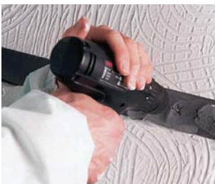
Figure 7.7 Textured coating being drilled through paste
