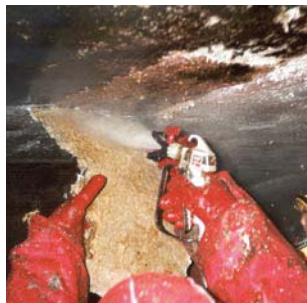
Figure 7.15 Spraying thin coating
