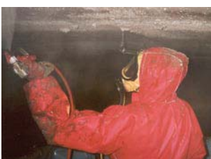
Figure 1.6 Controlled removal of asbestos
