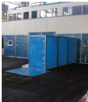
Figure 6.1 Enclosure with three-stage airlock
