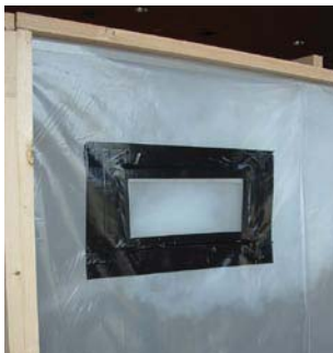
Figure 6.17 An enclosure being smoke tested
