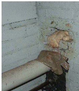
Figure 6.4 An enclosure sealed with expanding foam
