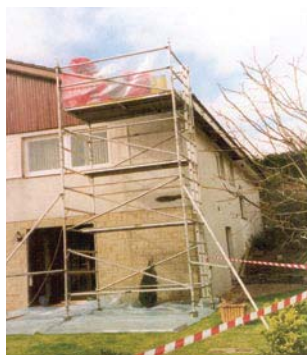
Figure 6.2 Work without an enclosure
