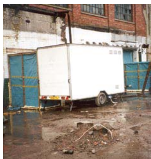
Figure 6.6 DCU attached directly to an enclosure
