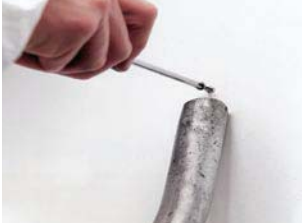
Figure 7.5 Shadow vacuuming during unscrewing of board
