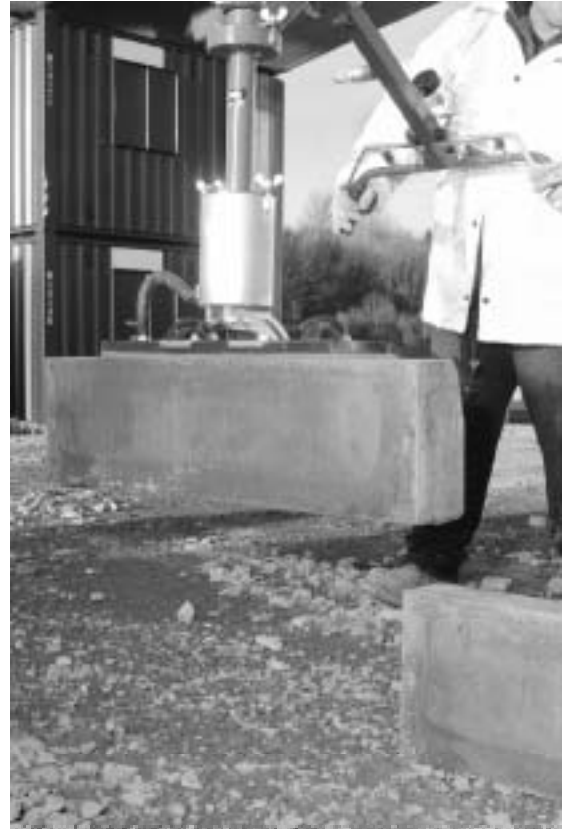
Figure 1 Handling kerbs using a vacuum lifter
