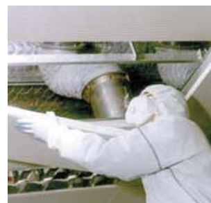
Figure 10 Removing panels to gain complete access for a Type 3 survey
