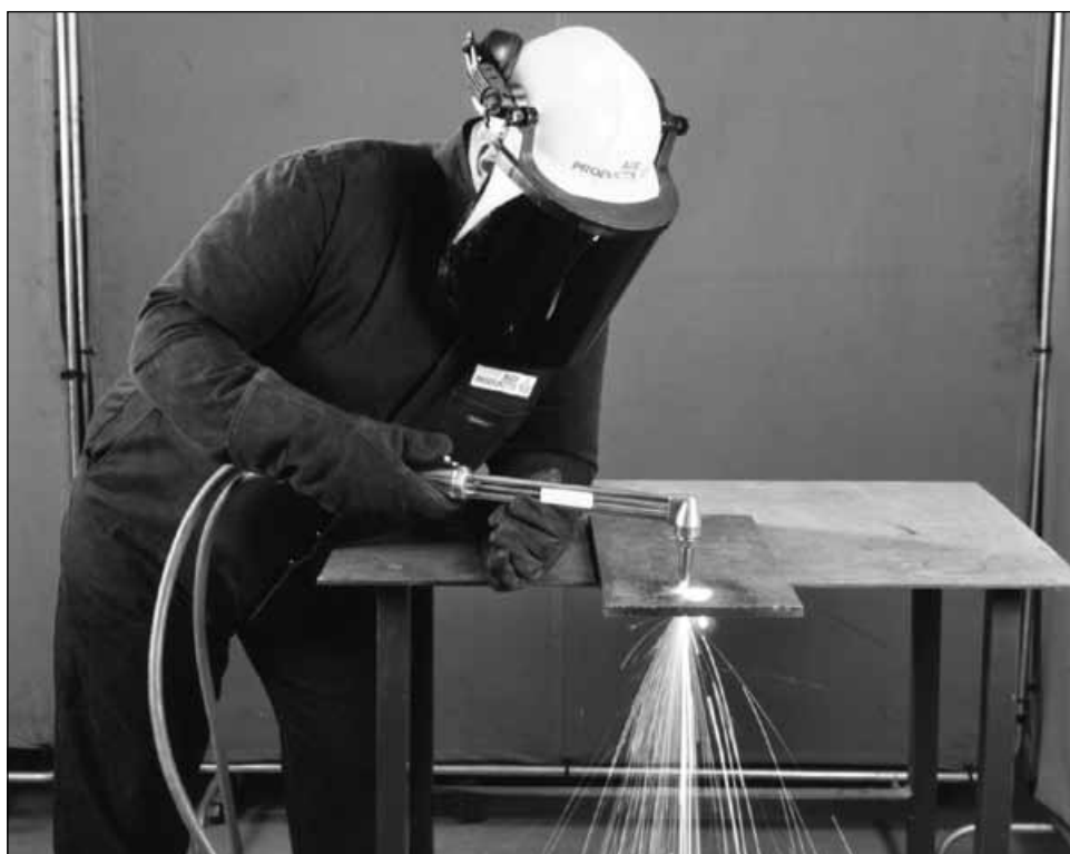
Figure 12 Flame cutting – use of protective equipment
