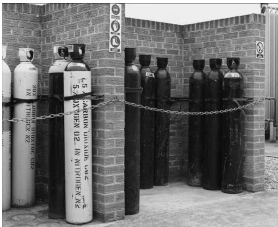
Figure 8 Storage of cylinders - fixed, upright in a well ventilated area
