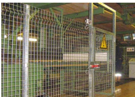
Figure 5 1.8 m perimeter fence and access gate with interlocked guard locking – this is the standard for new mechanised/automated lines
