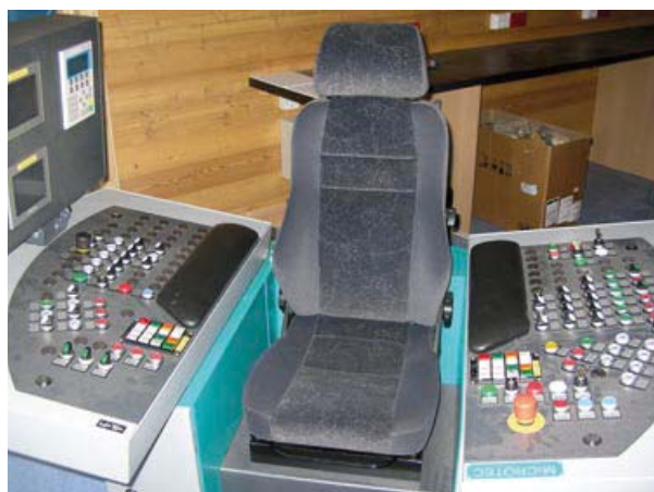
Figure 31 Automated sawmill control room
