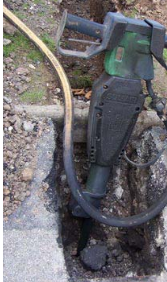
This charred breaker has struck an 11KV cable in a shallow trench
