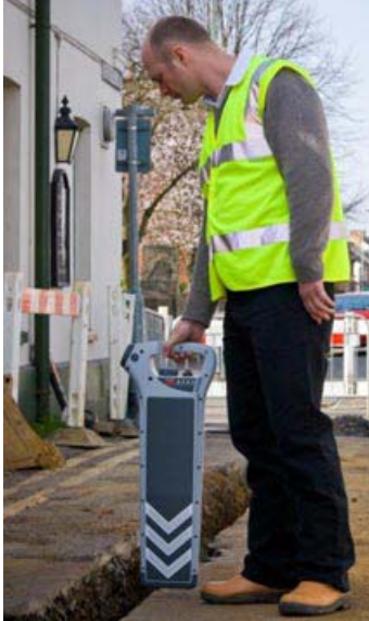
A cable avoidance tool in use
