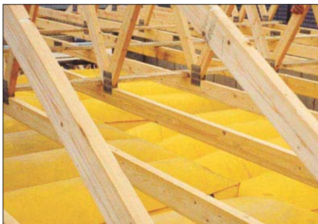
Figure 15(b) Air bags being used as a fall mitigation measure during roof work (Image courtesy of Airtex Safety Products Ltd)
