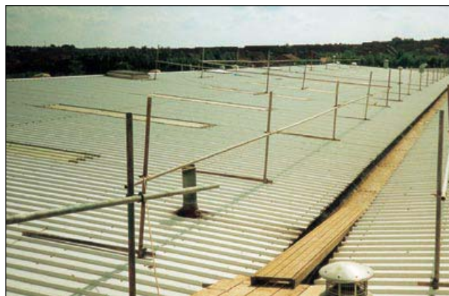
Figure 21 Demarcation barriers on a large, non-fragile roof, preventing access to the adjacent fragile roof lights. The roof lights are at least 2 m from the barrier
