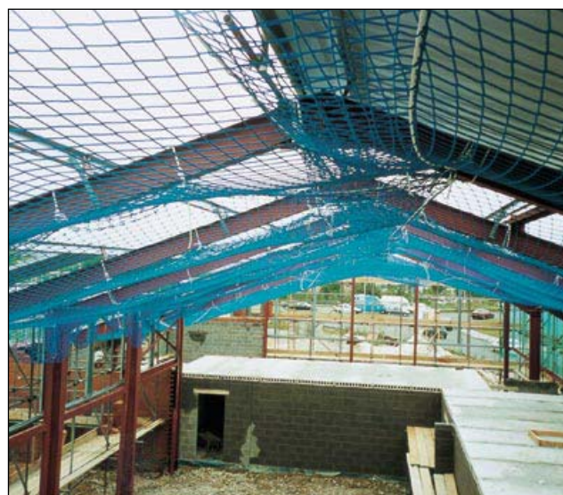
Figure 37 Use of safety nets during industrial roof work
