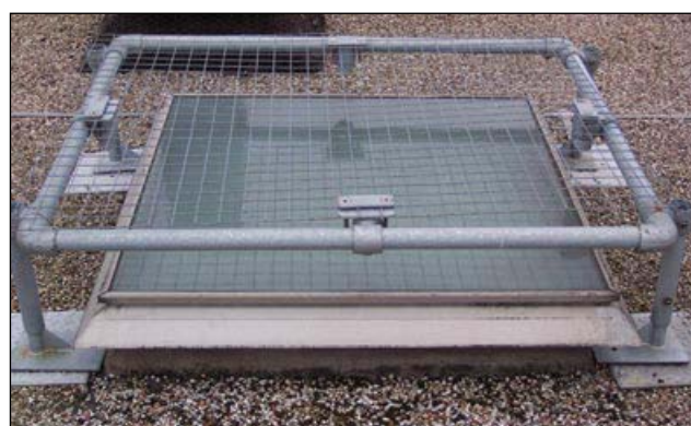
Figure 47 Galvanised mesh reinforcement between sheets of twin-skin roof light
