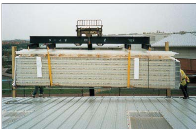
Figure 34 Delivering sheets to roof level onto the completed load-bearing section and behind the leading edge. (Note that the roof lights include mesh protection and are non-fragile)
