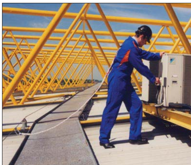
Figure 17 Work restraint harness used during short-term inspection on a flat roof (Image courtesy of Safesite Limited)
