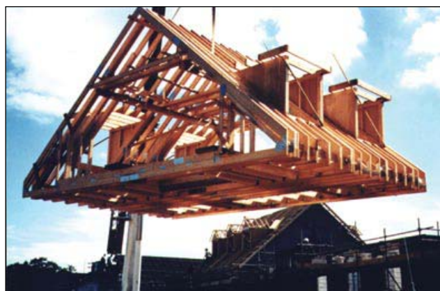
Figure 22 Craning a pre-assembled roof into position greatly reduces the need for work at height (Image courtesy of the Trussed Rafter Association)
