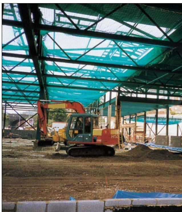
Figure 8 Debris netting used in addition to safety netting may enable work to be carried out safely below roof workers
