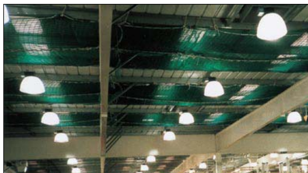
Figure 31 Safety netting used to provide protection for roof lights during minor roof works
