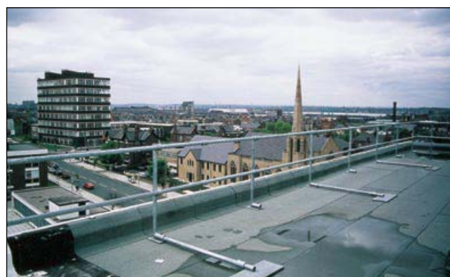
Figure 45 Permanent guard rail retrofitted during refurbishment work. Similar protection can be included in initial designs (Image courtesy of Safesite Limited)
