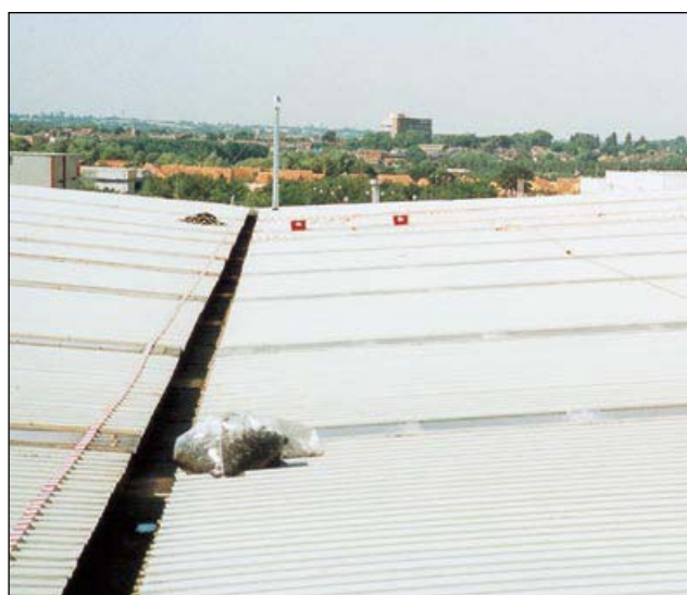
Figure 30 In some light conditions, it is difficult to distinguish the roof lights from the metal sheets on this type of roof. The valley gutter is very narrow and roof lights extend down to gutter level. Both of these features increase the risk during cleaning, maintenance or refurbishment
