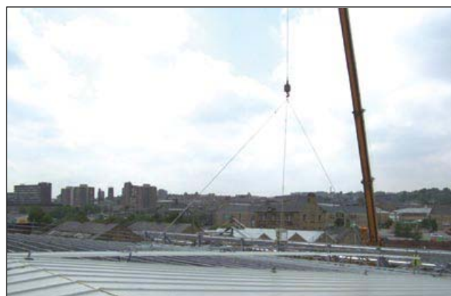
Figure 41 24 m long roof panels being mechanically lifted from ground level and installed on roof (a) (b) (c)
