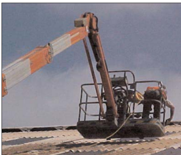
Figure 16 A mobile elevating work platform being used to replace a roof sheet
