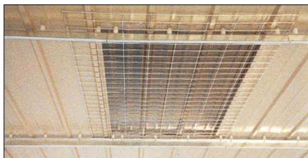
Figure 47 Galvanised mesh reinforcement between sheets of twin-skin roof light
