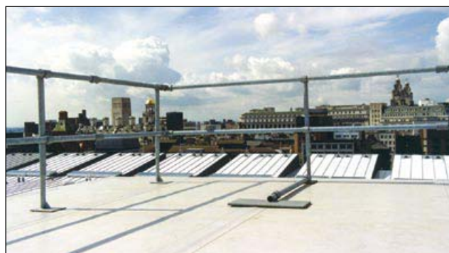
Figure 18 Temporary flat-roof edge protection. Adjustable supports enable work to progress with protection in place (Image courtesy of Safesite Limited)
