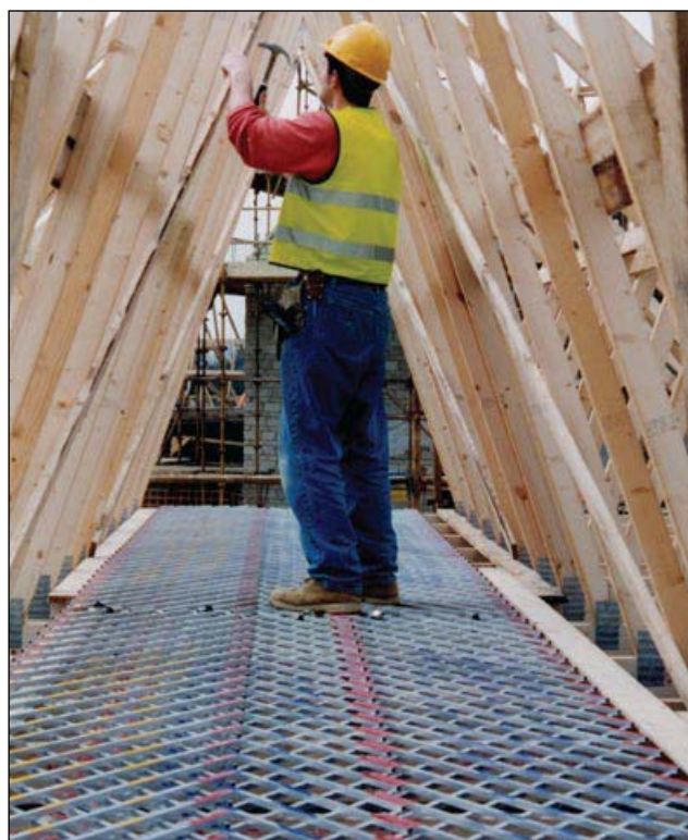
Figure 15(a) Decking system that provides a working platform in the roof eaves (Image courtesy of Oxford Safety Components Ltd)
