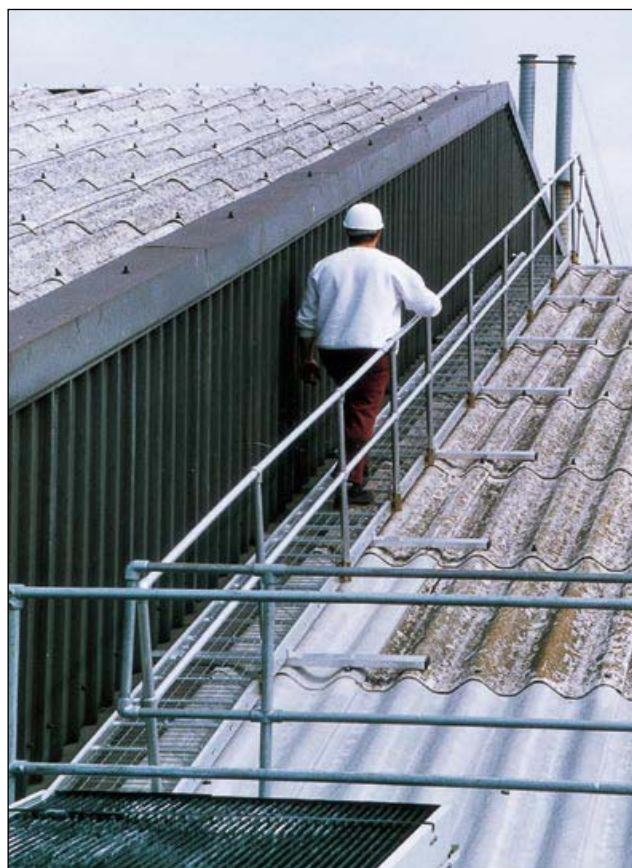
Figure 42 Permanent walkway giving safe access on a fragile roof. (This walkway was retrofitted, but similar access can be included in initial designs)
