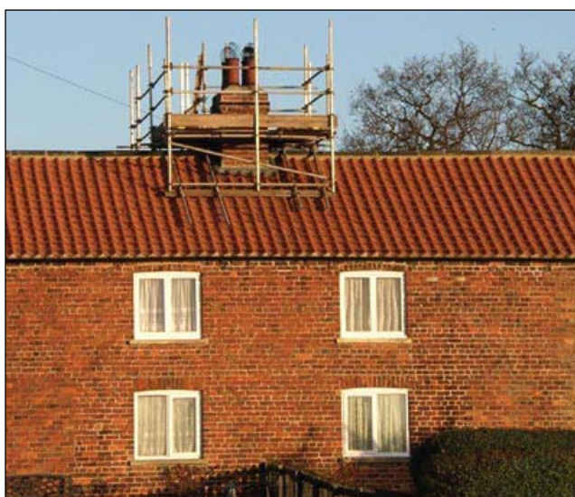
Figure 27 A traditional chimney scaffold
